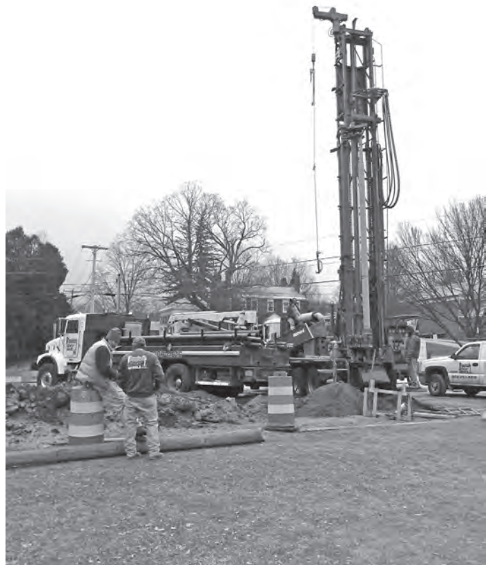
Parker Water Wells drills for water at the site of the new town hall.
